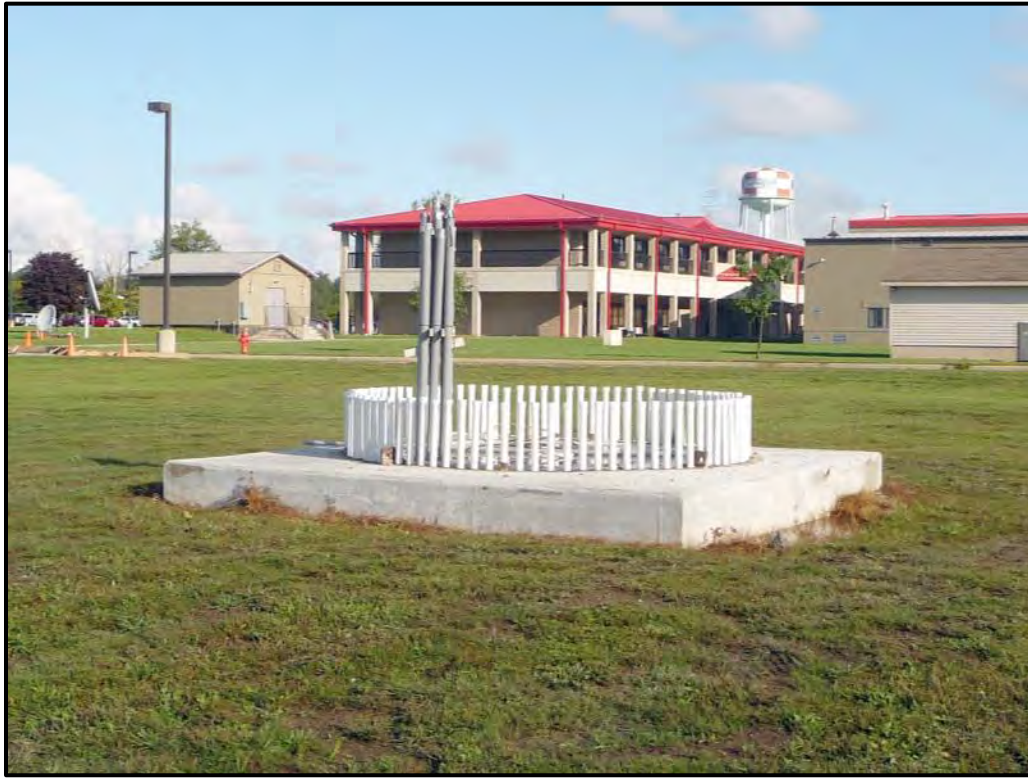
Photograph 2-1. Foundation for Proposed Wind Turbine at Camp Perry ANG
