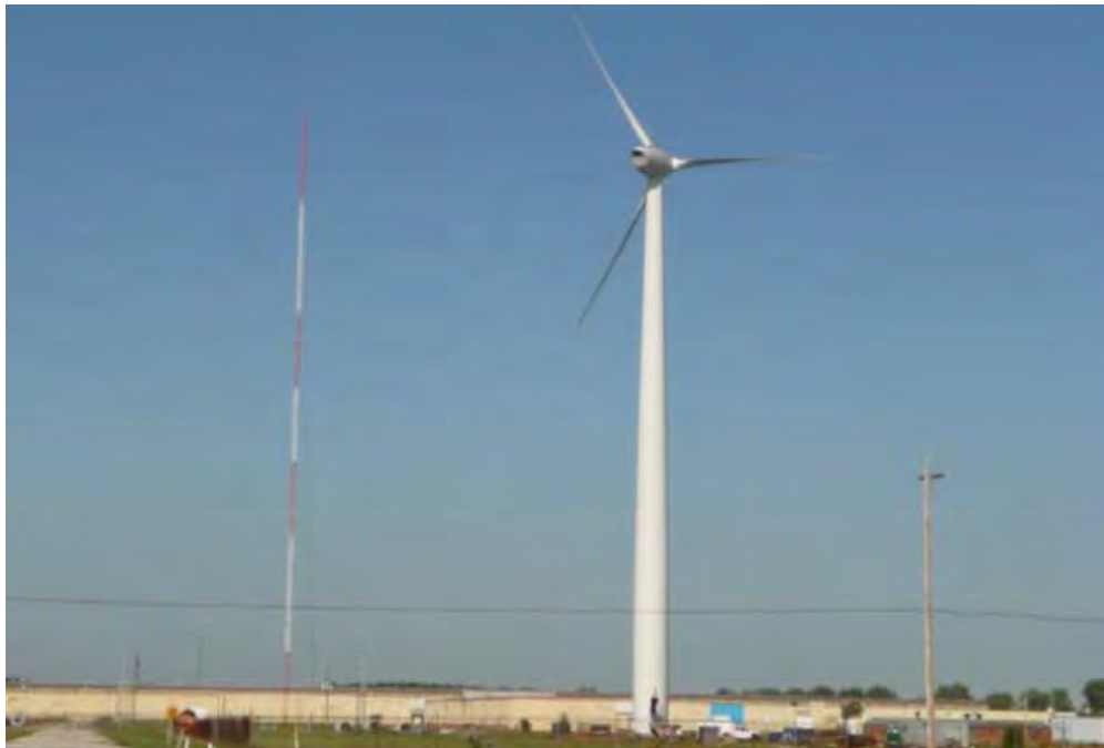
Figure 2.4. Photograph of a Single 600 kW Vestas 44 Wind Turbine at a Lake Erie Business Park
