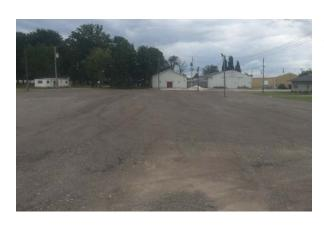
existing pavement and stabilized the sub-grade. Then, using the asphalt millings provided by the county, the airmen were able to spread, grade, and slope to implement a compaction plan that directed water shed and ensured proper drainage. In addition the airmen were able to utilize these millings to repair other vehicle area at the fairgrounds.
