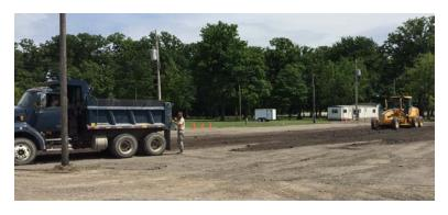
The main parking, roughly 37,400 square feet, consisted of poorly graded asphalt, which resulted in water penetration to the sub-grade and ultimately failure in multiple areas. Creating an eyesore and hazard with standing water, and ice in the winter. The RED HORSE team removed the
